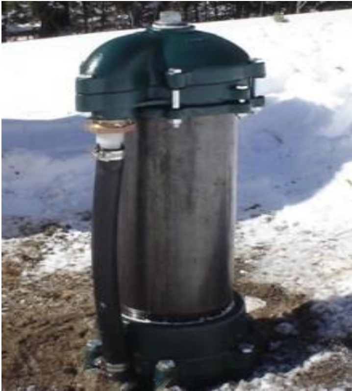
Typical wellhead with submersible pump
